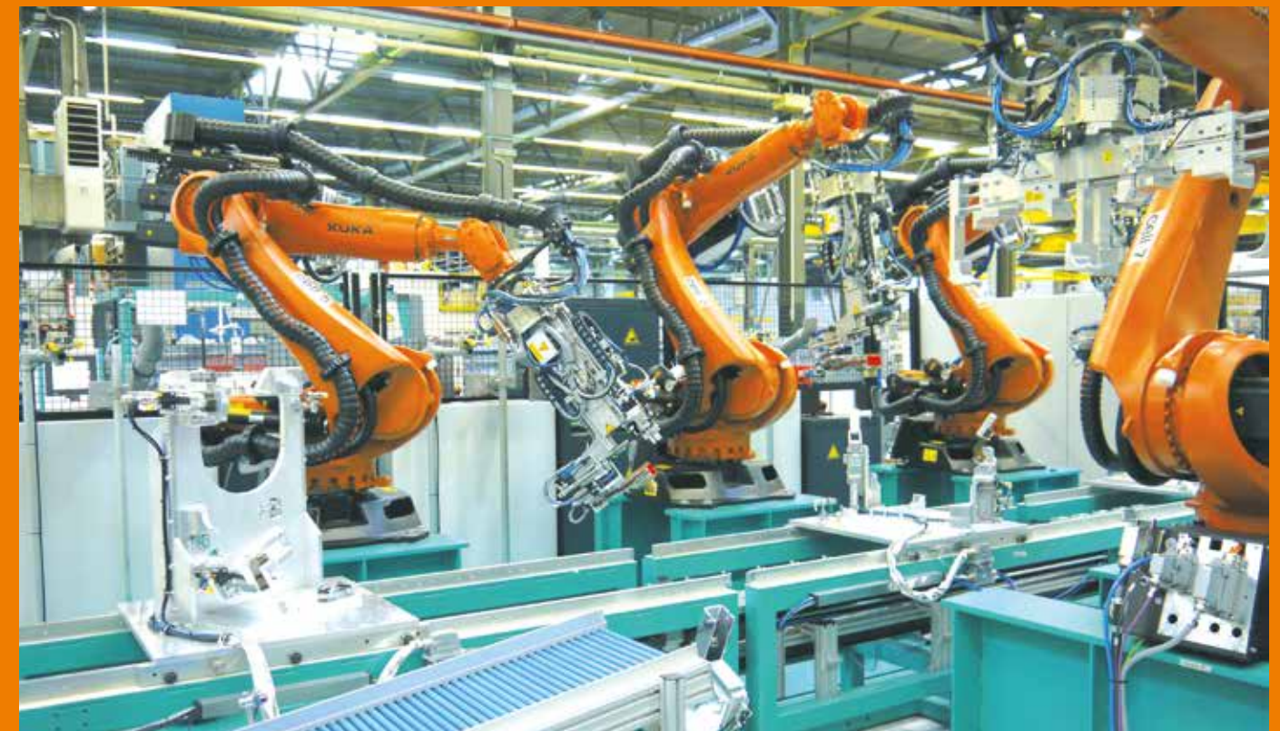
Flexible production - plant for the production of plastic vehicle tanks. In order to provide the end customer in the automotive industry with maximum flexibility, the production facilities are equipped completely with robots. The igus® RSP systems prevent loop formation of the e-chains® due to the multi-axis movements of the robot.
